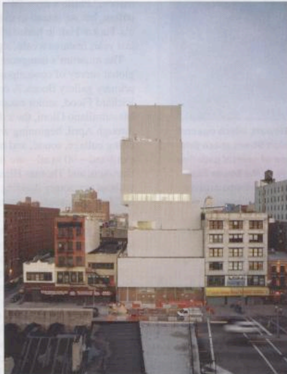
The New Museum's building, designed by the Tokyo-based architectural firm Sanaa, is an offset stack of six aluminum-mesh-clad boxes over a glass-enclosed lobby.
